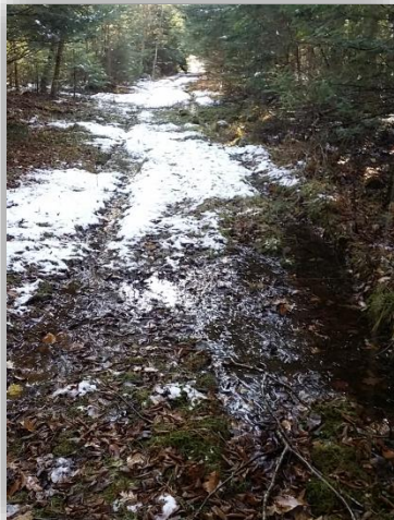
Water starts accumulating and running in the road about 1,000 feet before the stream crossing.
